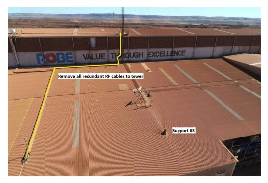
RF cables are to be removed from the roof to the equipment below. It is estimated there is no more than 20m of cables run in past the roof entry point which is accessible. Once cables are removed from roof the contractor is to reseal (water tight) the hole left by removed cables. Photos of sealed entry point to be taken on completeion.
